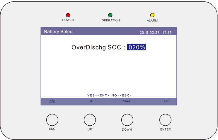
Figure 5.33 Over discharge SOC.
